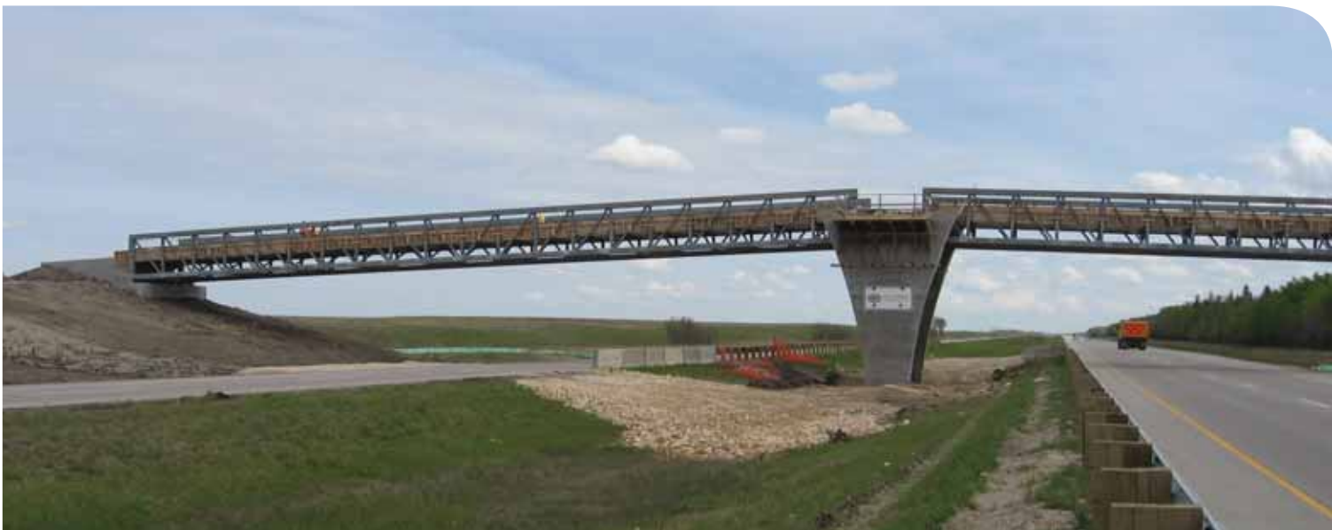
▲ A new pedestrian, bicycle and equestrian bridge across from the Birds Hill Provincial Park entrance lets people safely cross Highway 59.
